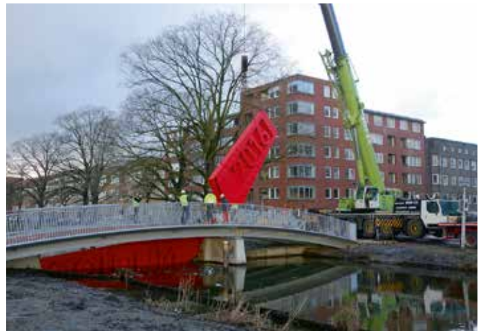
Montage deurdelen in funderingsdrager.
