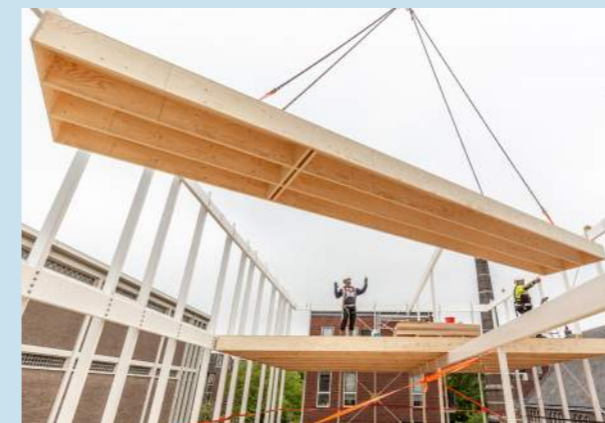
Figure 2: Wooden floors installation
