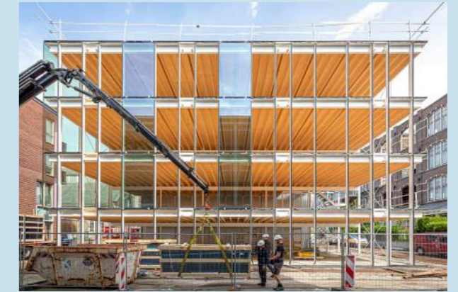
Figure 3: Glass facades installation
