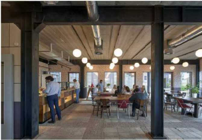
▲ FIGURE 3: REUSED STEEL IS KEPT IN SIGHT IN VARIOUS PLACES, SUCH AS IN THE RESTAURANT
