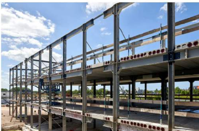
▲ FIGURE 4: CONSTRUCTION OF THE DONOR STEEL FROM THE GORLAEUS BUILDING
